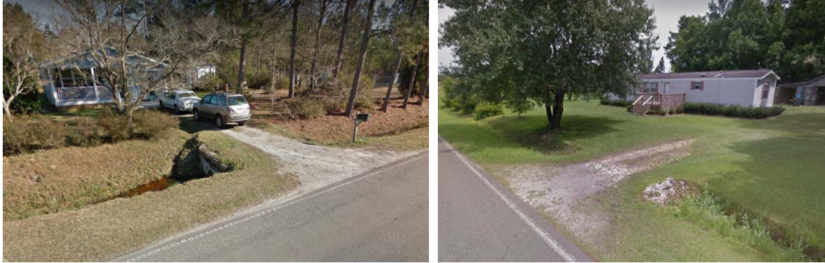
Narrow unpaved driveways over drainage ditches can pose a challenge to serving rural residences.
